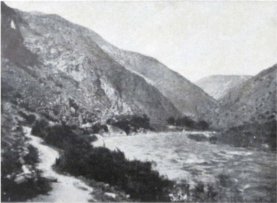
A VIEW ON THE TSCHOROCH
